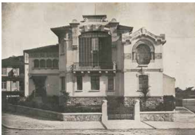
Fachada principal da casa/ atelier Malhoa (Achilles, 1909: Intercalar III).
